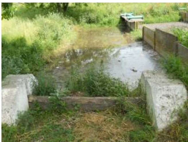
SEAU Corabia – detaliu “patari uscare namol”
