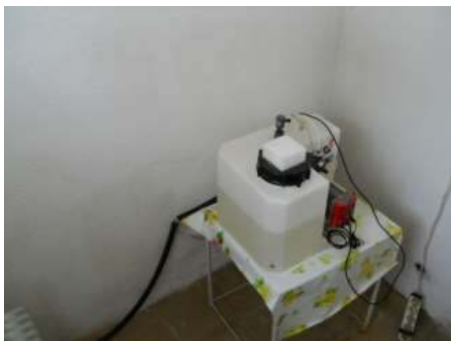
SP Re-pompare Corabia –clorinare a apei empiric
