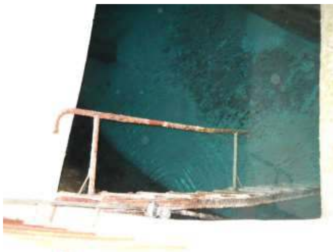
SP Re-pompare Corabia – accesul in sala pompelor
